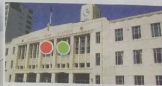
Central Fire Station, 2 Oriental Pde
